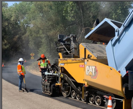
Loomis Arterial and Collector Pavement Repair
