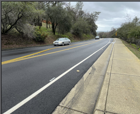
Auburn 2022 Street Overlay Project
