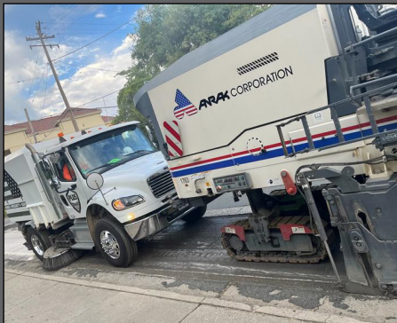
Auburn 2023 Street Overlay Project
