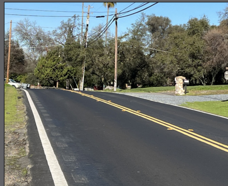
Laird Road Asphalt Rubber Chip Seal Project
