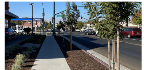
- Lincoln Boulevard streetscape improvements and repaving
